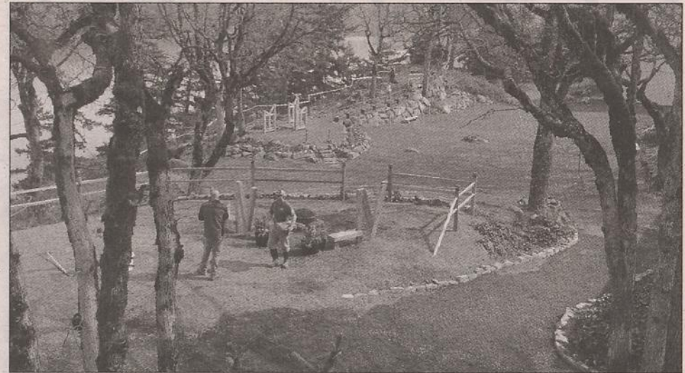
The wedding venue, the broad lawn on the Vagabond's north side, gets finishing touches on April 3. Below, owner Grant Polson stands at the location in this November 2013 photo.
