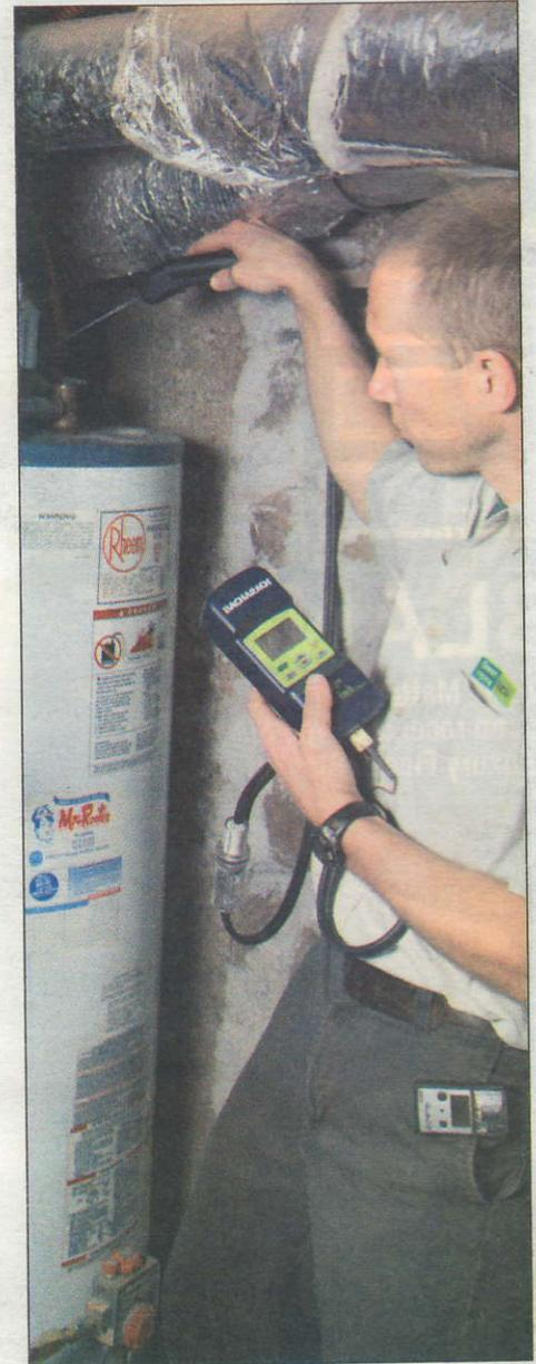
**Dana Scheffler, Green Home Construction weatherization technician, conducts energy audits and indoor air quality assessments with the help of computer read-out mechanical technology. Once leaks are located, remedies may include duct sealing and insulation. When tightened up and properly ventilated, an effective thermal envelope of a home can reduce energy waste considerably and increase owner comfort within the home.**
